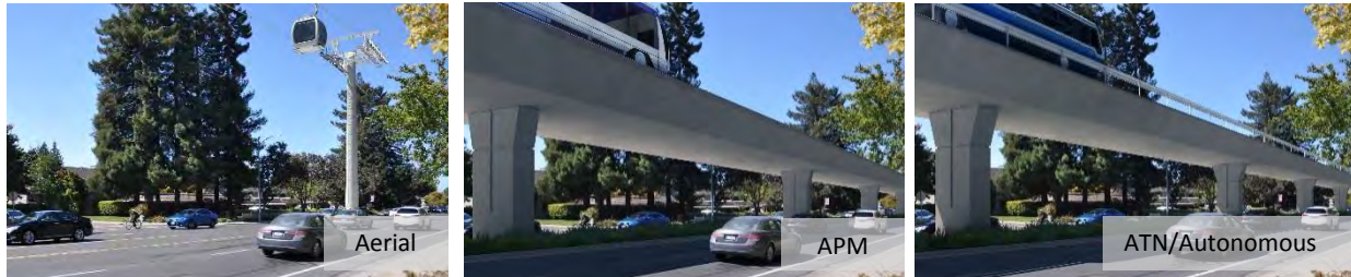
Figure 8-1 Aerial, APM, and ATN/Autonomous Transit Infrastructure
