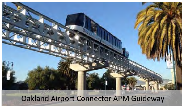
Figure 8-3 Example APM Guideway Infrastructure
