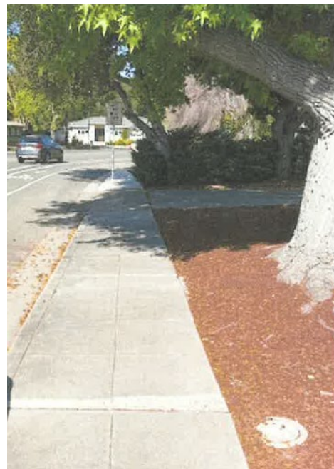
Figure 3 and Figure 4: Photos Showing the Proximity of Tree to Sewer Cleanout, Sidewalk, and Existing Damage that Will Need to Be Repaired
