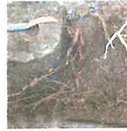
FIGS 10,11,12): Considerable amount of work has been done to expose roots in support of this appeal. Front view of the pool equipment shed area shows how the deep roots have begun to surface making their way underneath the slab to the open area, where water is often available.
