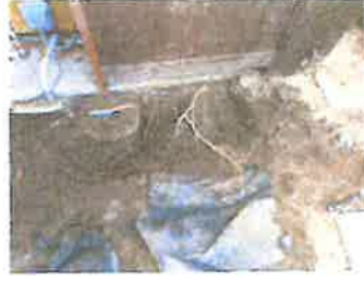
FIGS 10,11,12): Considerable amount of work has been done to expose roots in support of this appeal. Front view of the pool equipment shed area shows how the deep roots have begun to surface making their way underneath the slab to the open area, where water is often available.
