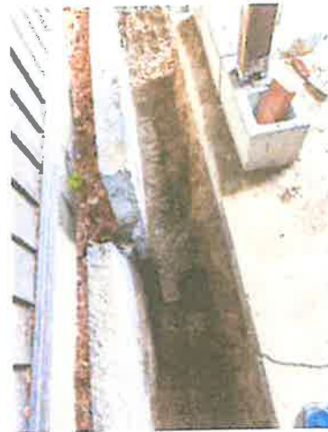
FIG 1: Top view of fence showing proximity to tree. FIG 2: Other side showing foundation damage already caused. Pool equipment sits on the concrete slab, and shows the start of a crack on the bottom right. Current estimated cost of repairs is $15,000.
