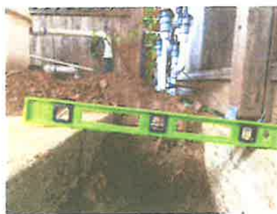
FIG 5: Concrete slab where pool equipment is at 240 Chatham Way. The property line retaining wall on the right is the property ground level. Level shows the elevation change caused by the redwood tree roots uplifting the ground underneath the slab.
