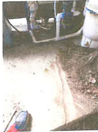
FIG 7: Proximity to pool equipment with crack extending precariously underneath the plumbing and pumps. Repairs estimated at $15,000.
