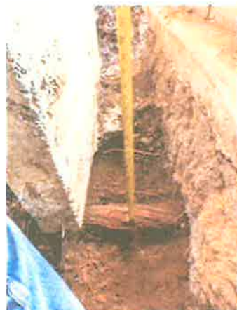
FIG 3: 4" inch root found 24" directly below the concrete footing of the property line retaining wall ( FIG 4 ), which has been uplifted nearly 2' by the roots.
