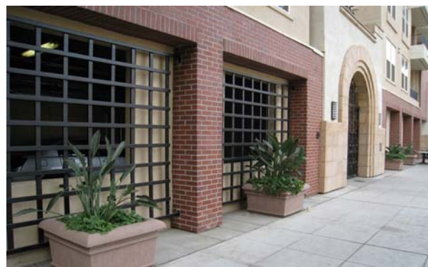
A structured podium garage with screening
