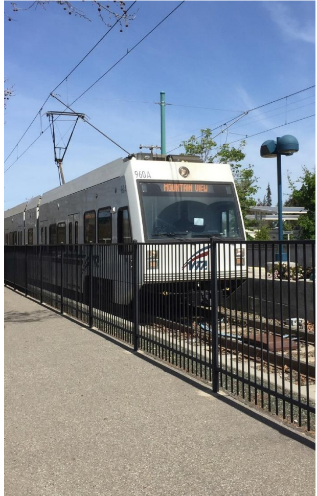
Middlefield Light Rail Station
