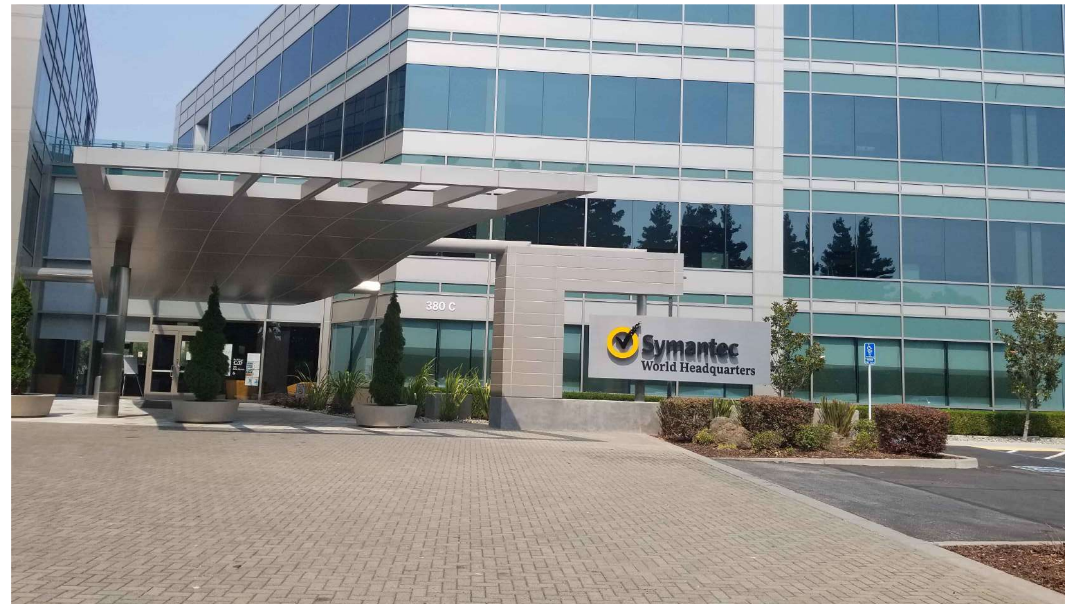
1 EXISTING PHOTO @ BUILDING C/D MAIN LOBBY
