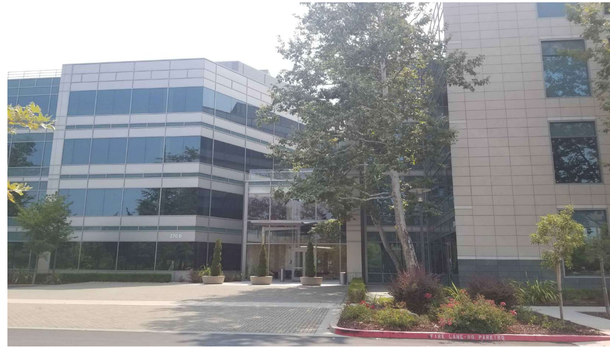
2 EXISTING PHOTO @ BUILDING A/B COURTYARD LOBBY
