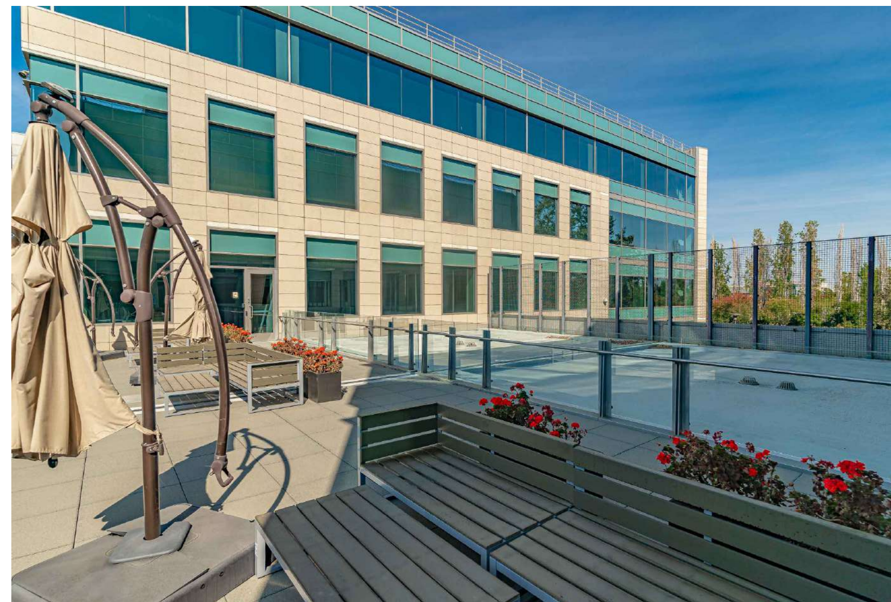
3 EXISTING PHOTO @ BUILDING C/D THIRD FLOOR ROOF TERRACE
