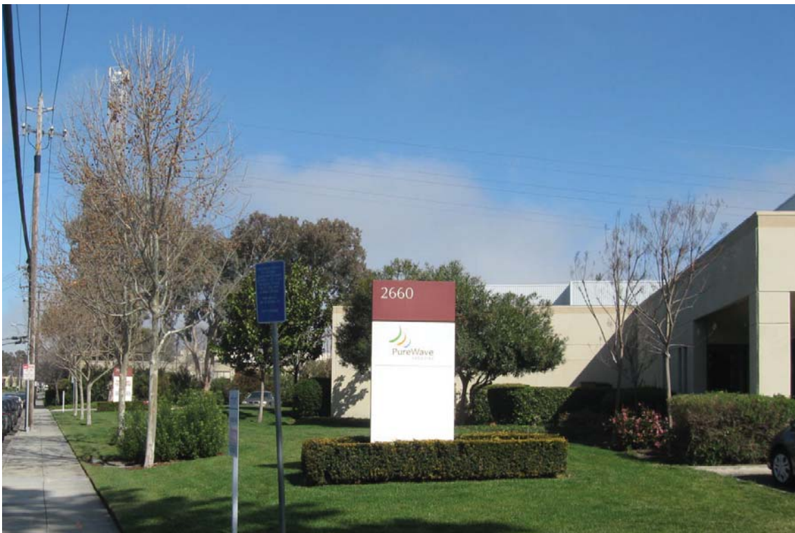
PHOTO 8: Building at 2660 Marine Way, view to the northeast.
