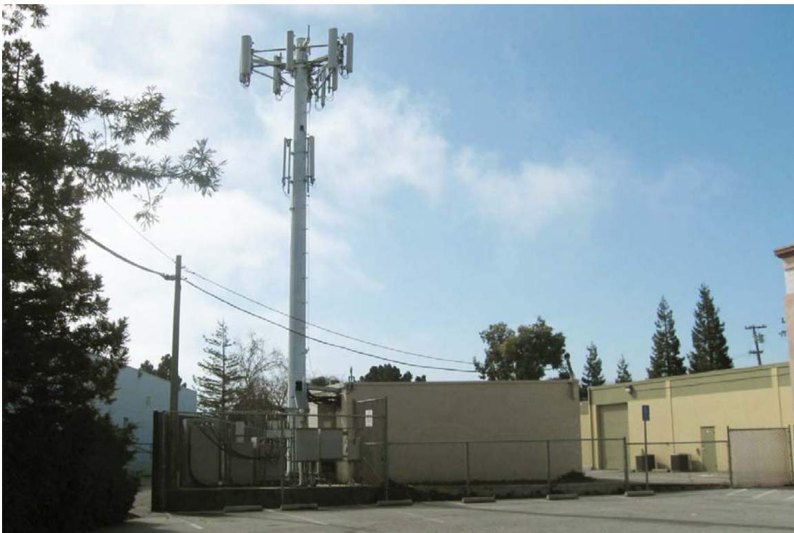
PHOTO 2: Cell tower at 2634 Bayshore Parkway, view from the Garcia Avenue sidewalk towards the southwest.
