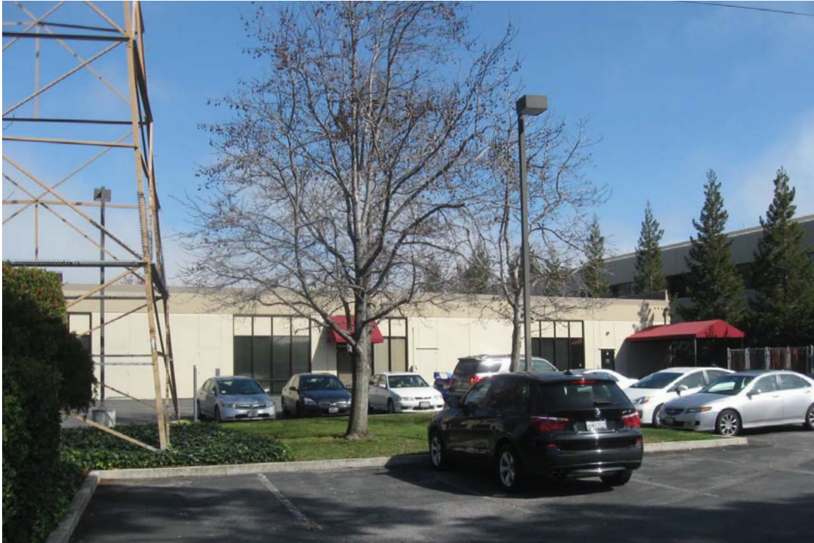
PHOTO 3: View of 2698 Marine Way, with PG&E power line structure in the foreground. View towards the northeast from sidewalk of Marine Way.
