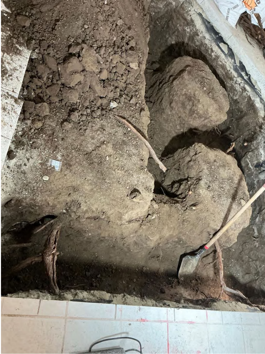
West Side Roots. Perimeter is Trenched
