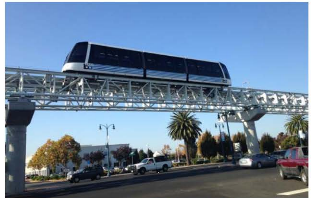
Doppelmayr Cable Car: Cable Liner (Oakland, CA)
