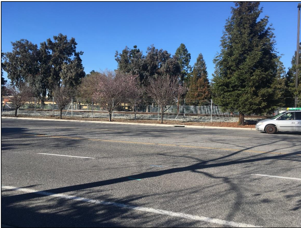
Photograph 6: Caltrain tracks across East Evelyn Avenue north of the project site, facing north
