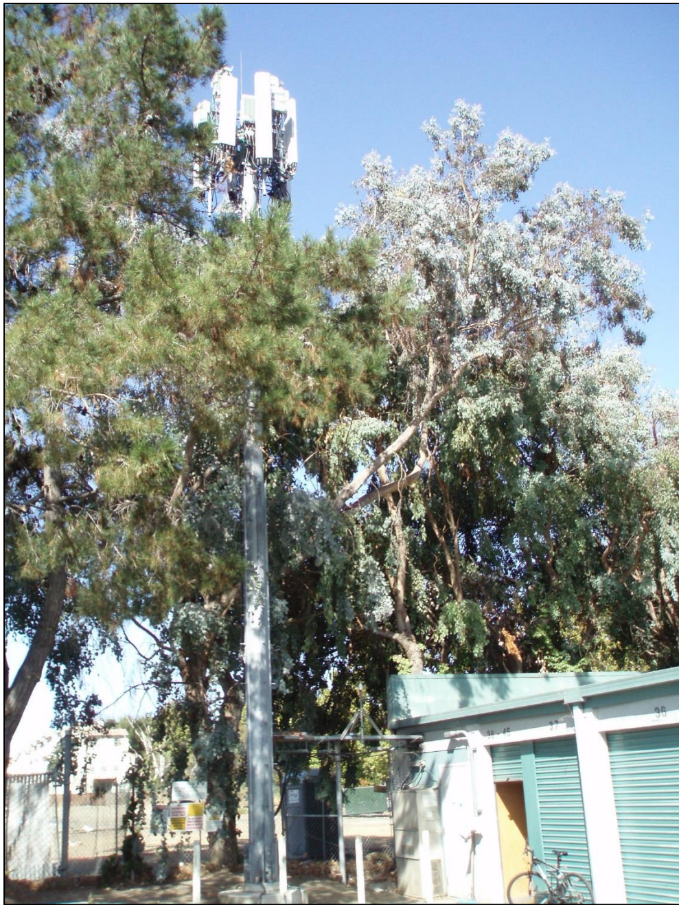
Photograph 5: Existing on-site wireless communications antenna and associated equipment to the left
