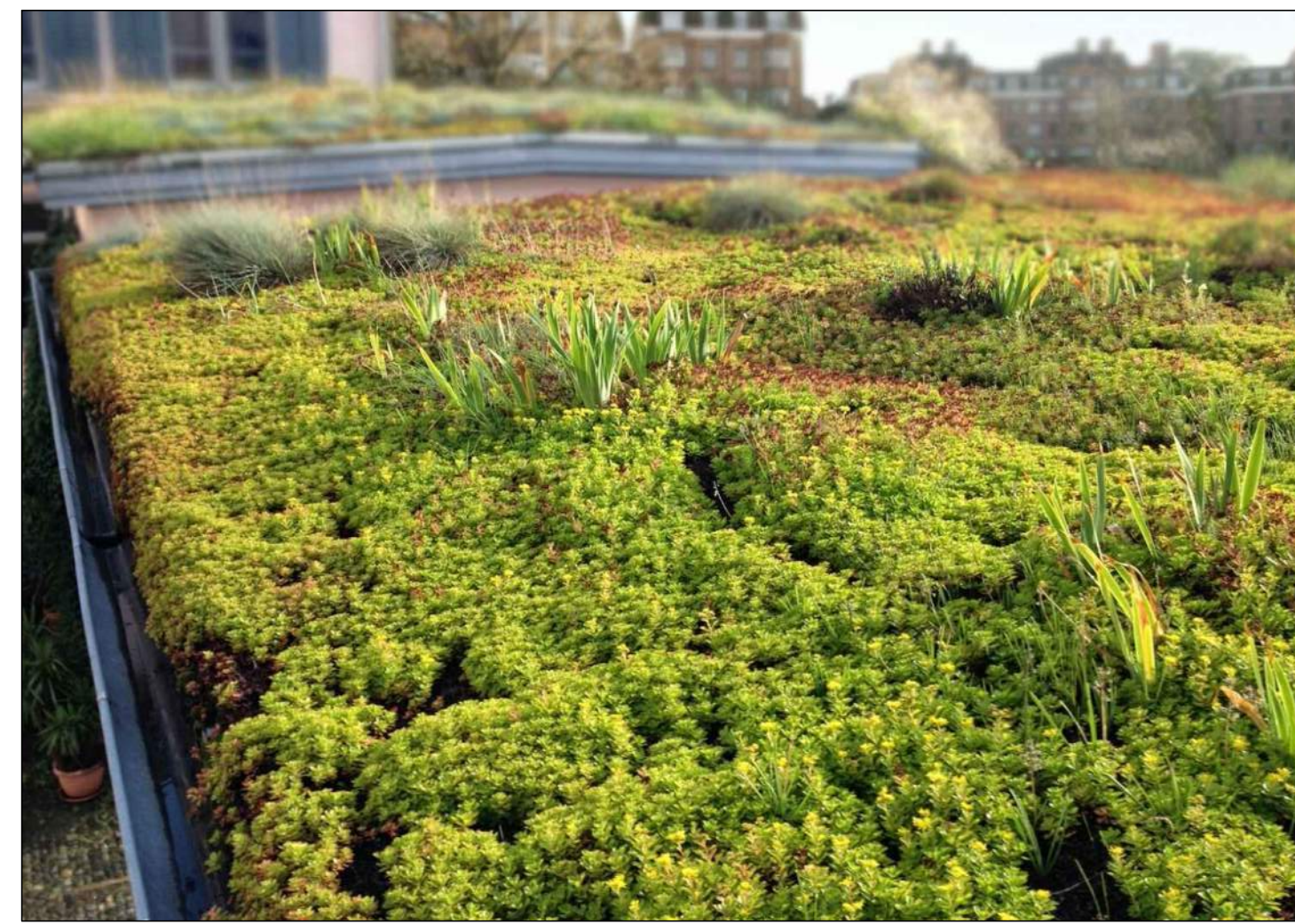
6 Extensive Green roof Sedum Mat NTS
