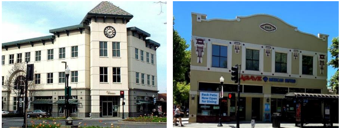
Fig. H.26: Building roof forms fronting Castro Street should reinforce the character of the historic commercial buildings with flat roof forms, parapets, cornices and decorative details.
