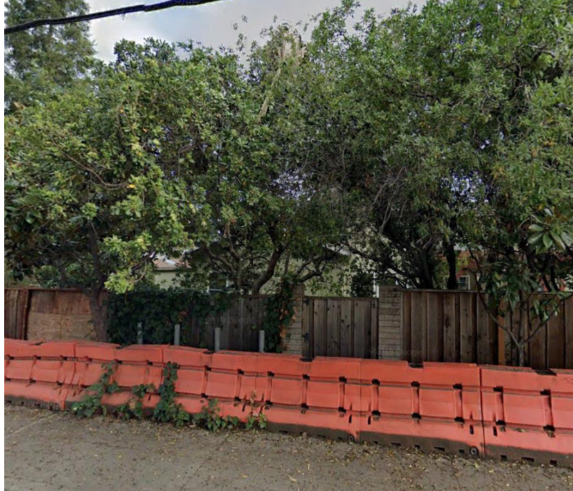
Figure 4 – Temporary Barrier System at Grant Road/South Drive
