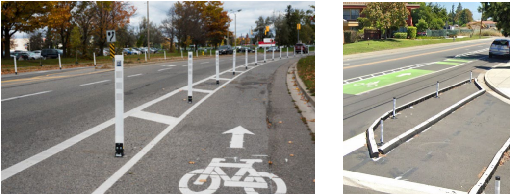
Figure 4: Example Delineators and Rubber Curbing
