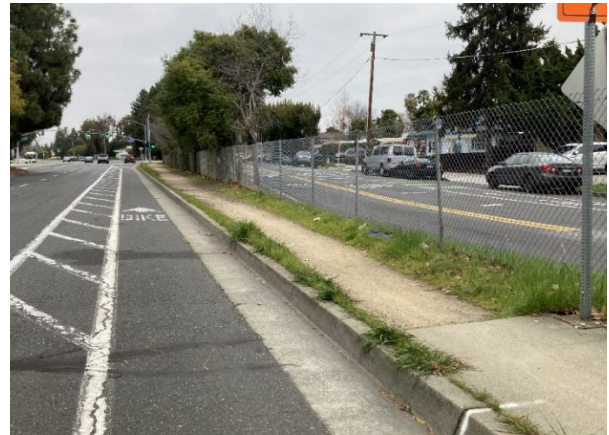
Figure 3: Sidewalk Gap Looking North
