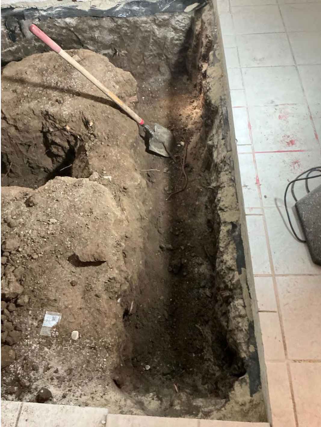
Clean cuts for Root Pruning. Perimeter is Trenched
