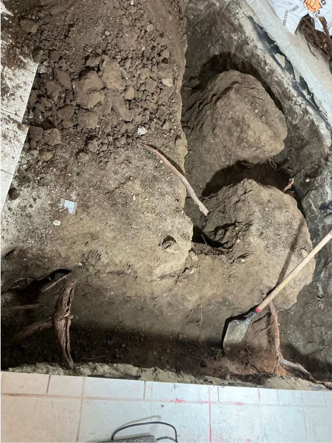
West Side Roots. Perimeter is Trenched
