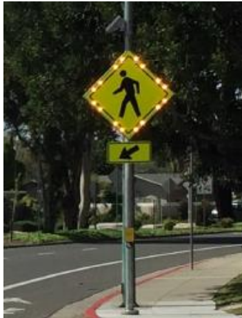
Figure 3 – Example of LED-Enhanced Pedestrian Crossing Sign
