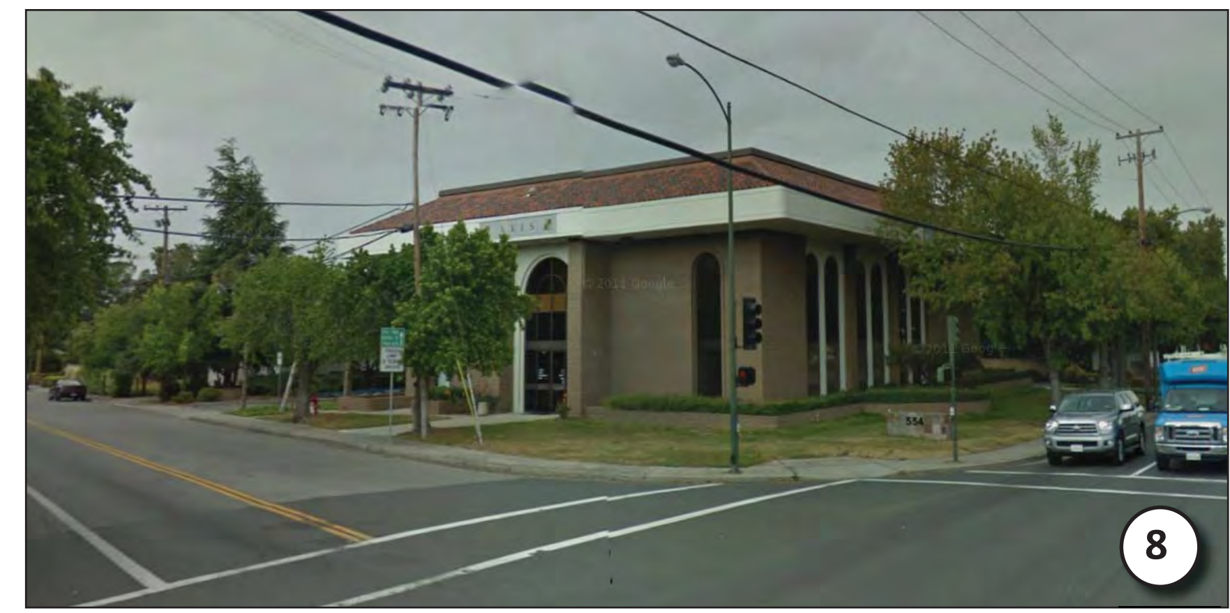
VIEW WEST ON FAYETTE AND SAN ANTONIO INTERSECTION
