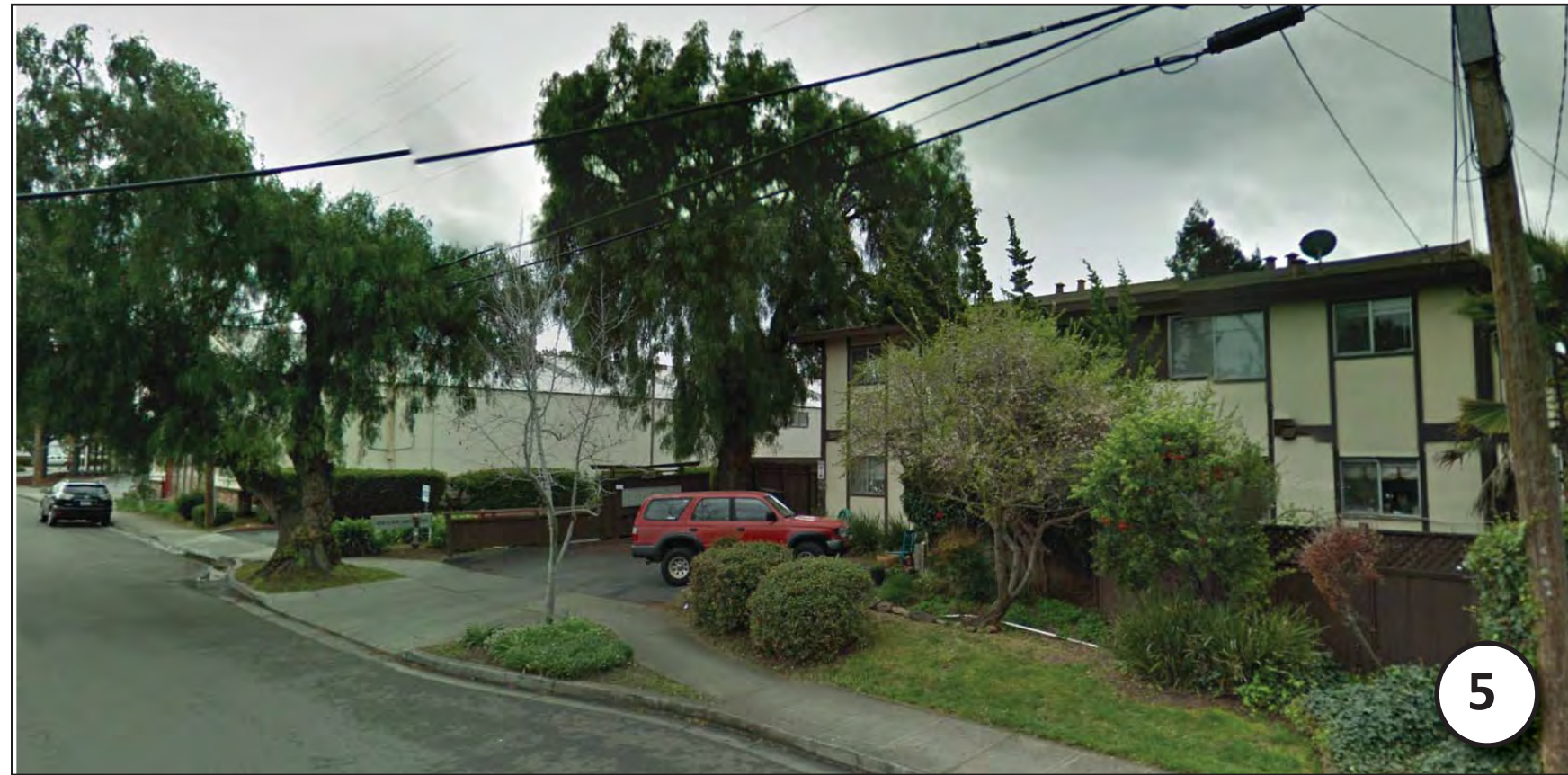
VIEW SOUTH ON MILLER AVE
