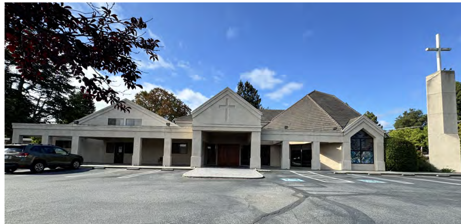
CHURCH MAIN ENTRANCE 4
