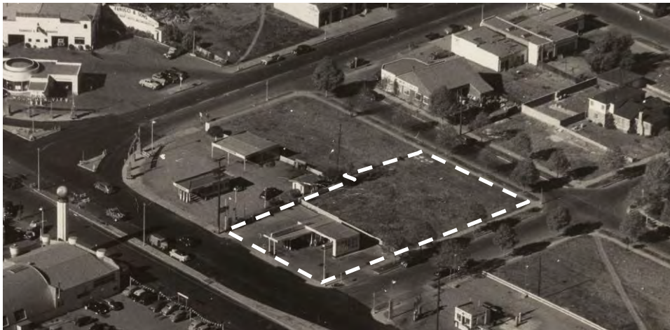
Figure 2. Birds-eye aerial view of subject property (approximate current boundary in white) ca. 1950-1955 (Mountain View Public Library 1950-1955).
