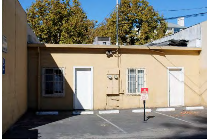
Photograph 2. Rear (east) exterior, viewed from alley at rear of building, facing west.
