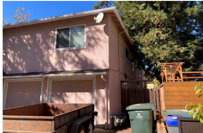
Photograph 5 Oblique view of north exterior along the north property line, facing west-southwest
