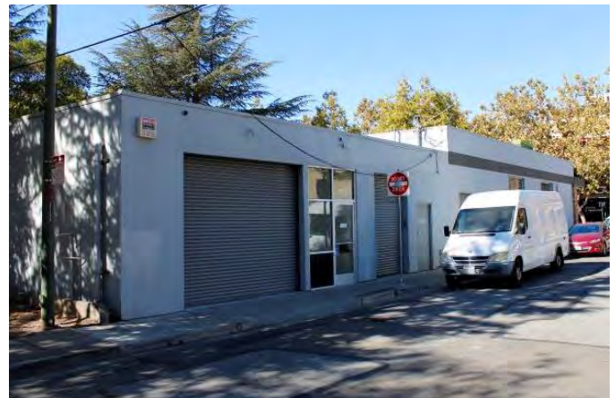
Photograph 7. North exterior along Fairmont Avenue, facing southwest.
