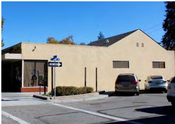
Photograph 4. South exterior, viewed from Castro Street and Fairmont Avenue, facing north.
