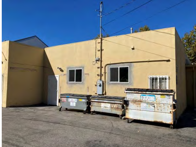
Photograph 2. Rear (east) exterior, viewed from alley behind building, facing southwest.
