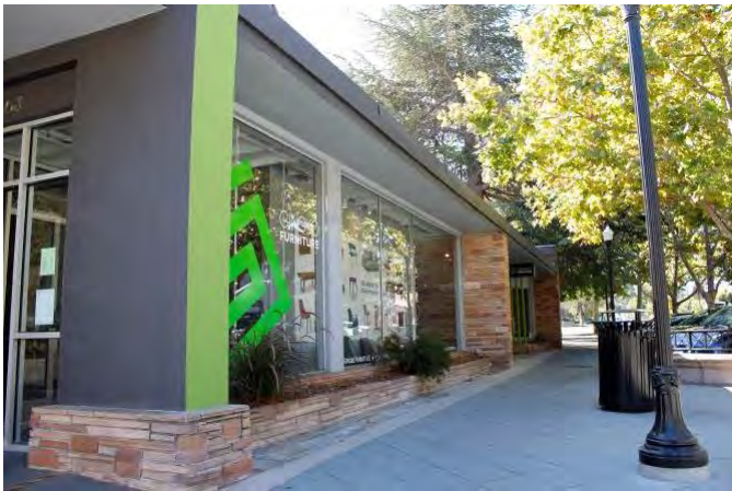
Photograph 4. Oblique view of façade, facing south.
