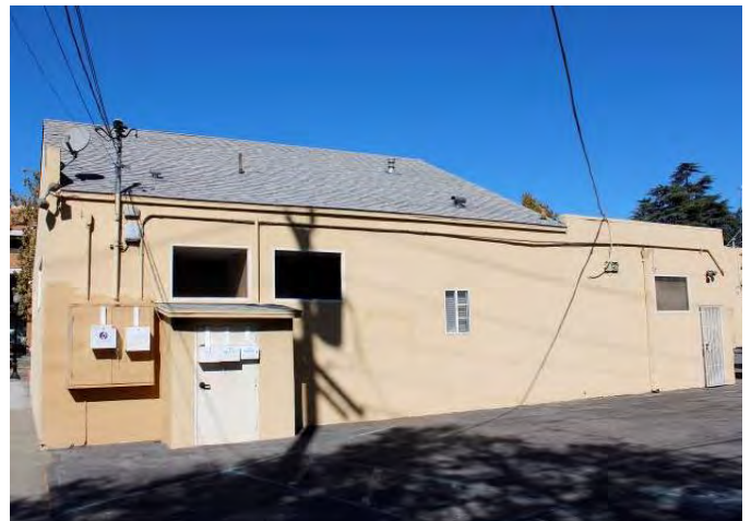
Photograph 5. Rear exterior, viewed from alley, facing west.
