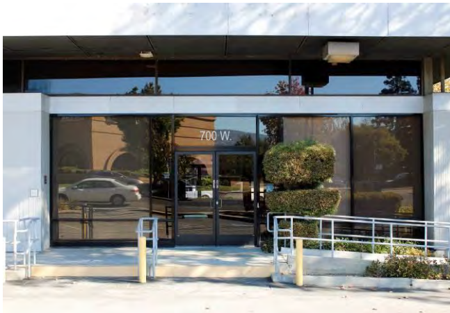
Photograph 3. Storefront and concrete ramp at main entrance, facing north
