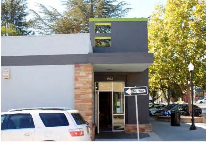
Photograph 2. Entrance at northwest corner and pilon element above canopy, facing south.
