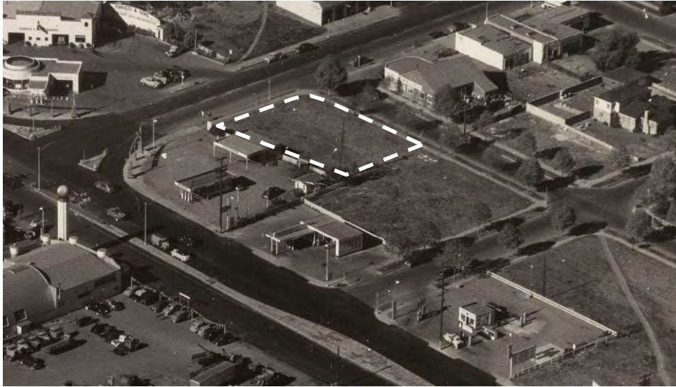
Figure 2. Birds-eye aerial view of subject property (approximate current boundary in white) ca. 1950-1955 (Mountain View Public Library 1950-1955).
