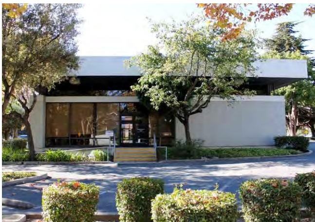
Photograph 5. Rear (north) exterior, facing south
