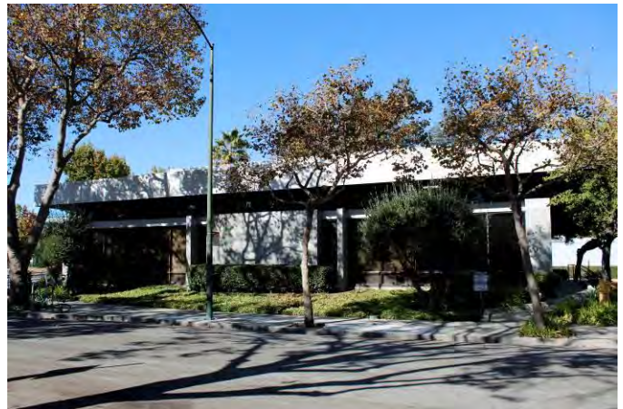
Photograph 4. East exterior viewed from Hope Street, facing southwest
