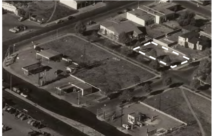
Figure 3. Birds-eye aerial view of subject property (approximate current boundary in white) ca. 1950-1955 (Mountain View Public Library 1950-1955).
