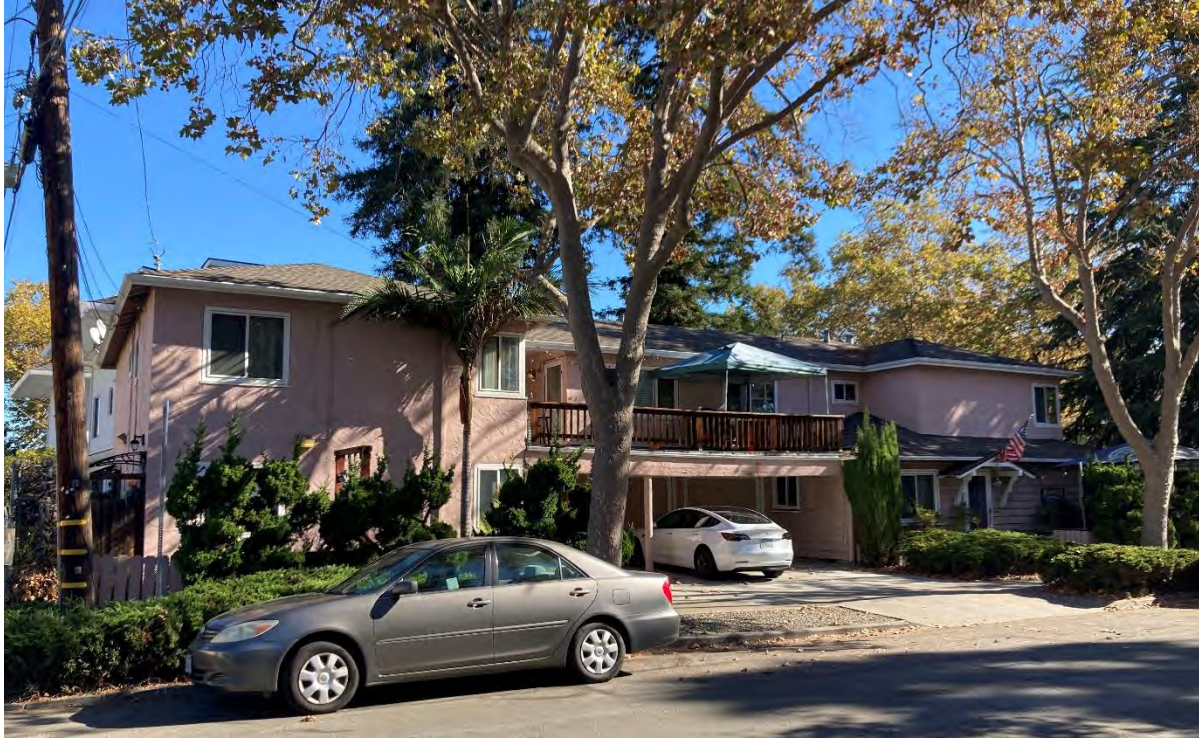
Photograph 3. 750 Fairmont Avenue, Camera Facing Northwest
