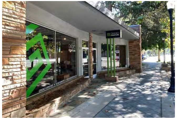
Photograph 5. Recessed entry and three-pole column beneath canopy, view facing southeast.
