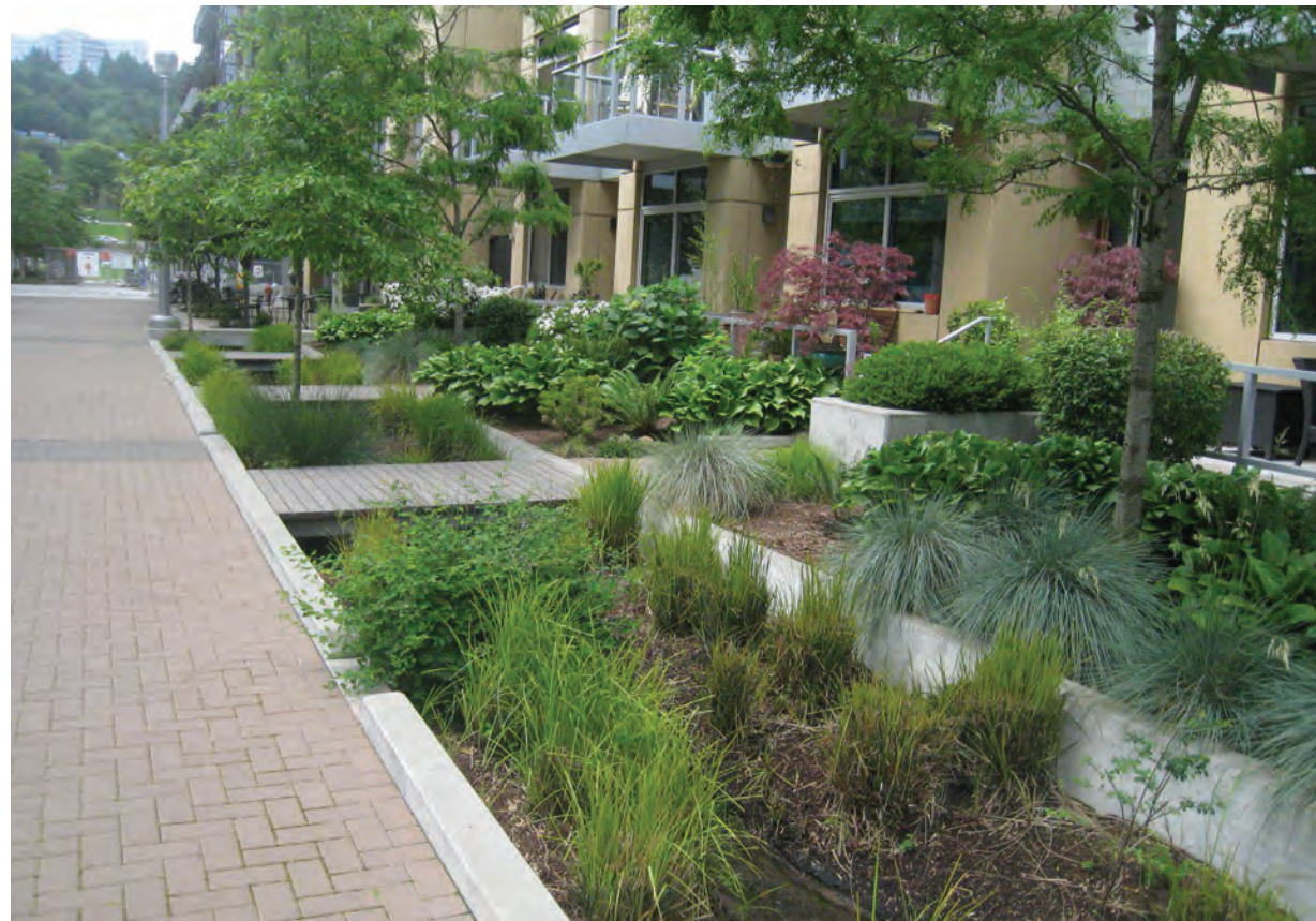
BRIDGES AT STORMWATER PLANTERS
