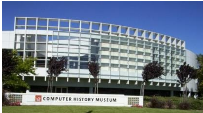
Landmark Entry Building
