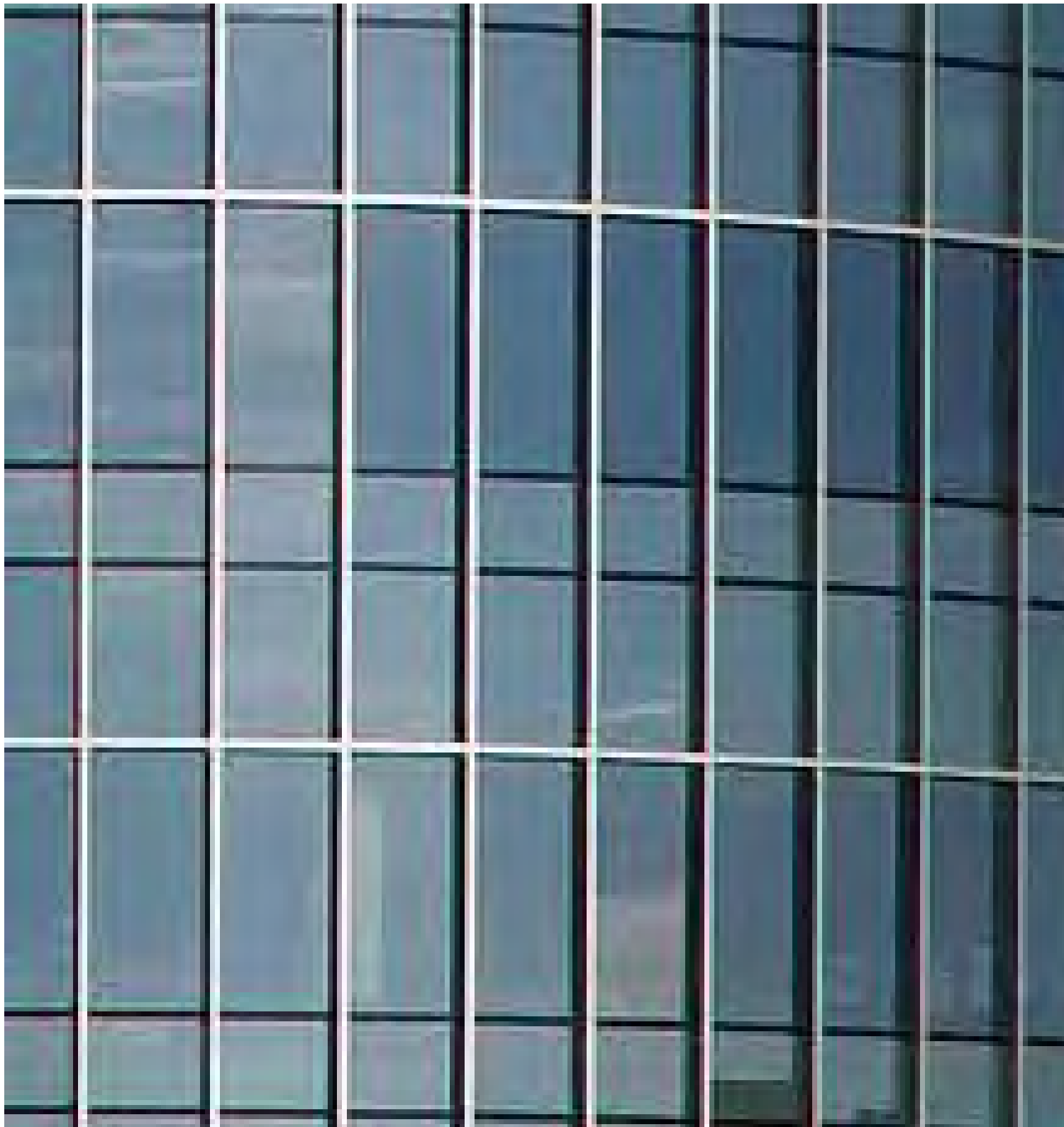
ALUMINUM FRAMED CURTAIN WALL WITH SPANDREL GLASS PANELS
