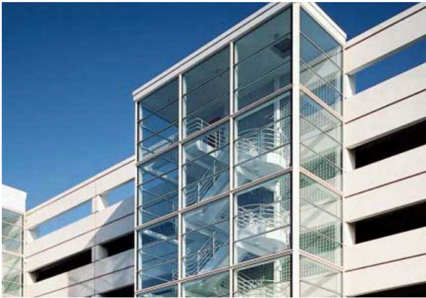
PARKING - GLASS STAIR TOWERS ON WEST SIDE AND TYPICAL PRECAST CONCRETE SPANDREL
