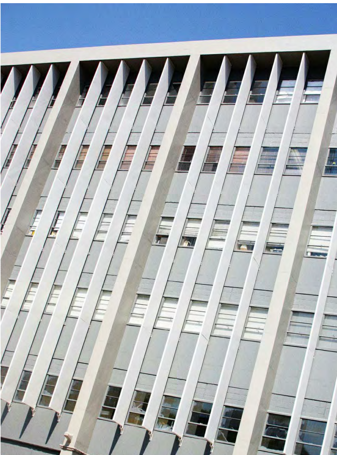
VERTICAL SUNSHADES ON WEST FACADE
