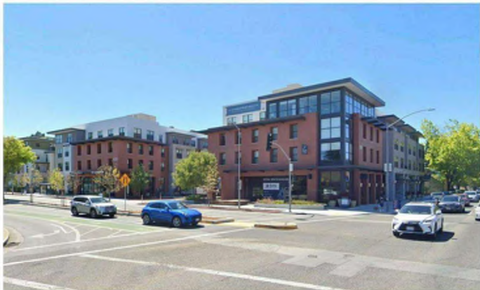
1. APARTMENT @ CASTRO ST & ECR INTERSECTION
