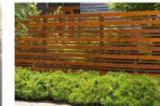
Wood Screen Fence
