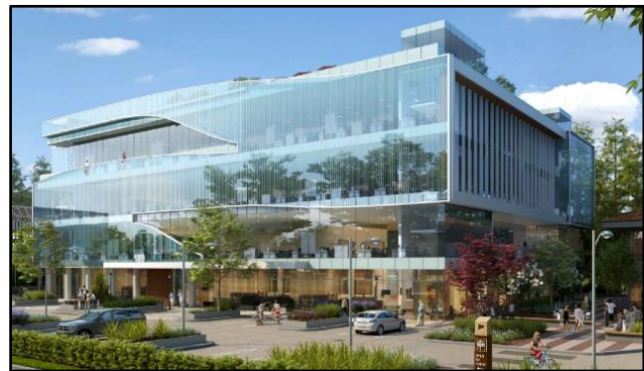
Figure 6: View from North
