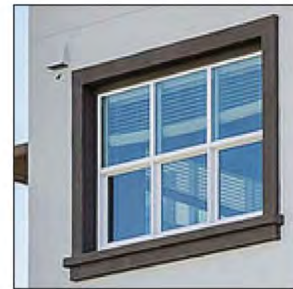
7 ENHANCED BUILDING TRIM SMOOTH PLASTER OVER FOAM
