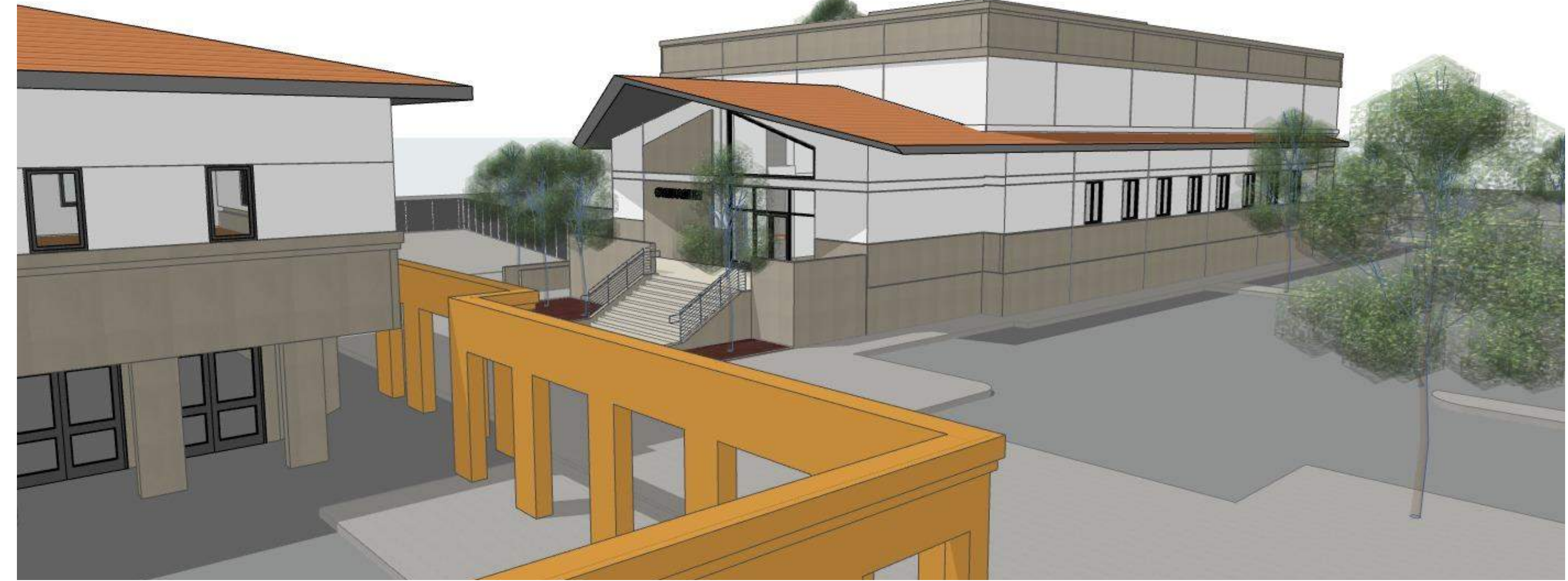
2 EAST SIDE ALONG PARKING LOT
