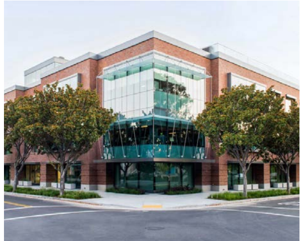
High-quality facade with interesting materials, windows, and articulation
