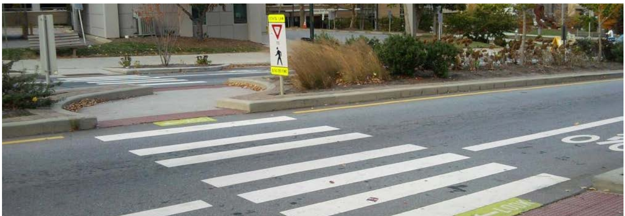
Example of mid-block crosswalk
