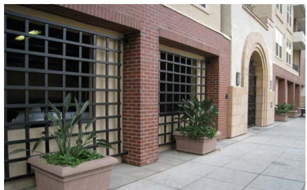
A structured podium garage with screening
