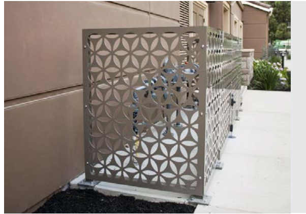
Decorative screening to minimize the appearance of utilities
