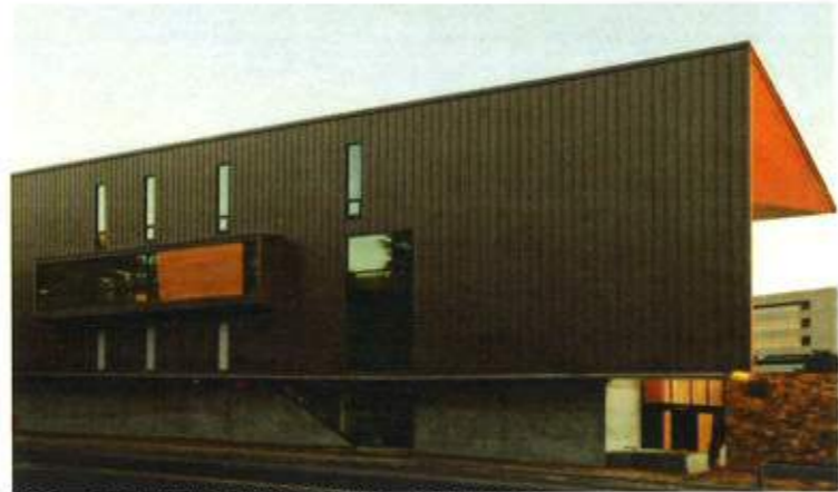
11 A5.1 STANDING SEAM SIDING - COLOR D
