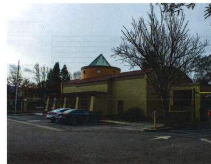
3 A0.1 VIEW FROM REAR OF SITE
