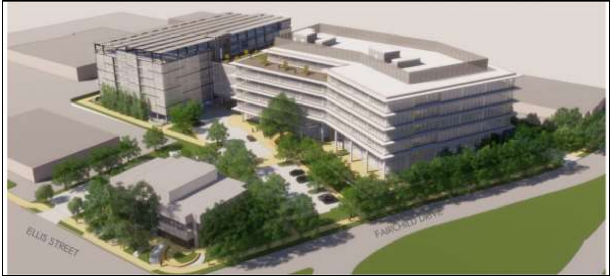
Figure 4: View from Northeast
