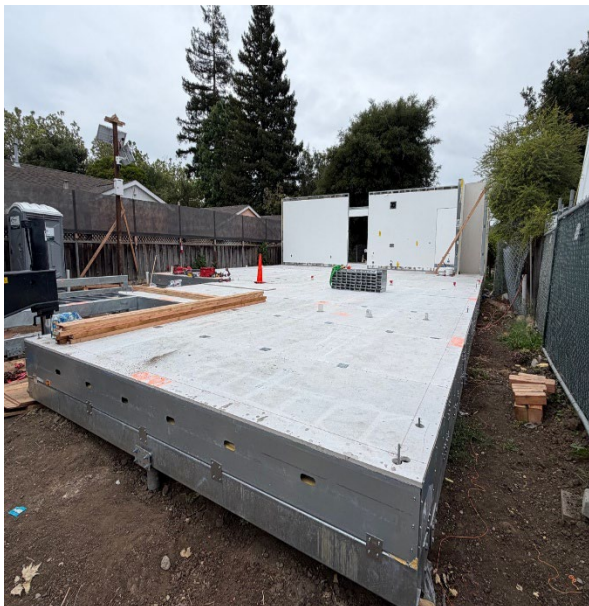
Photo #7 Photo of home construction panels
