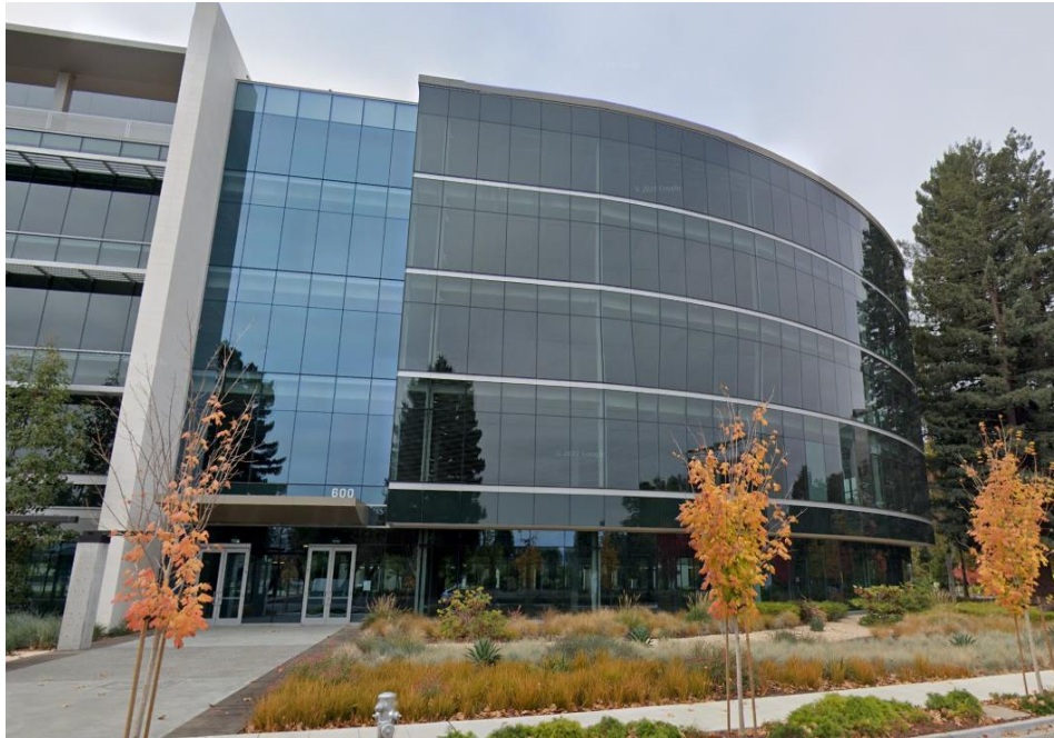
Glass Curtain Wall
