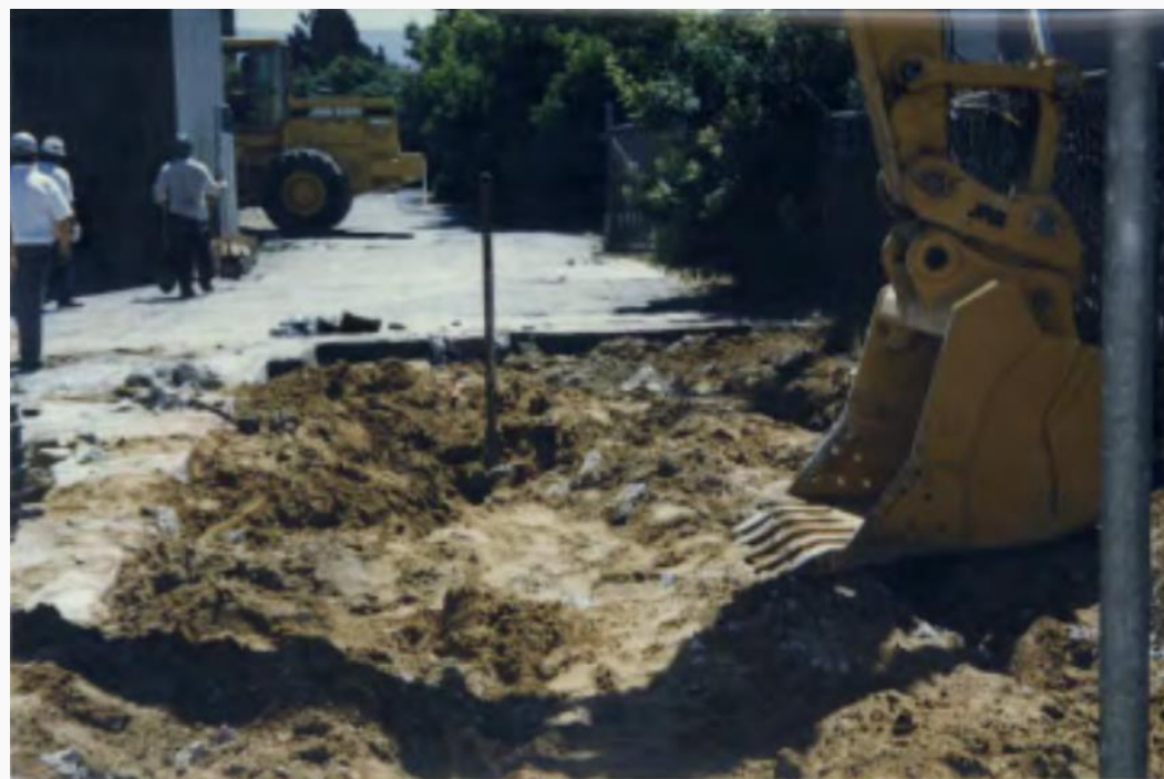
Contaminated soil excavation
