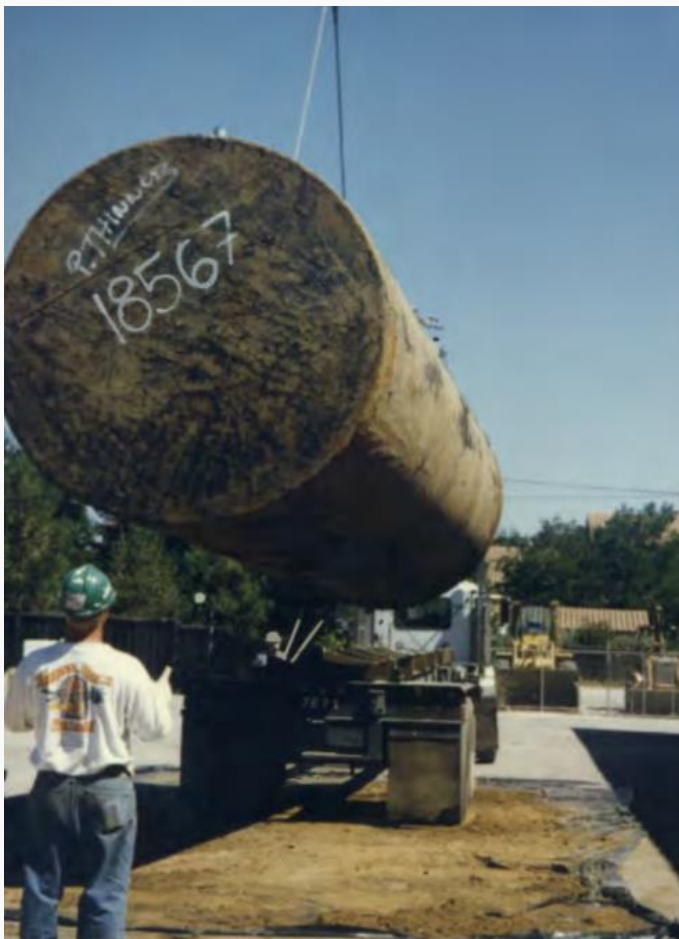
Underground Storage Tank removal
