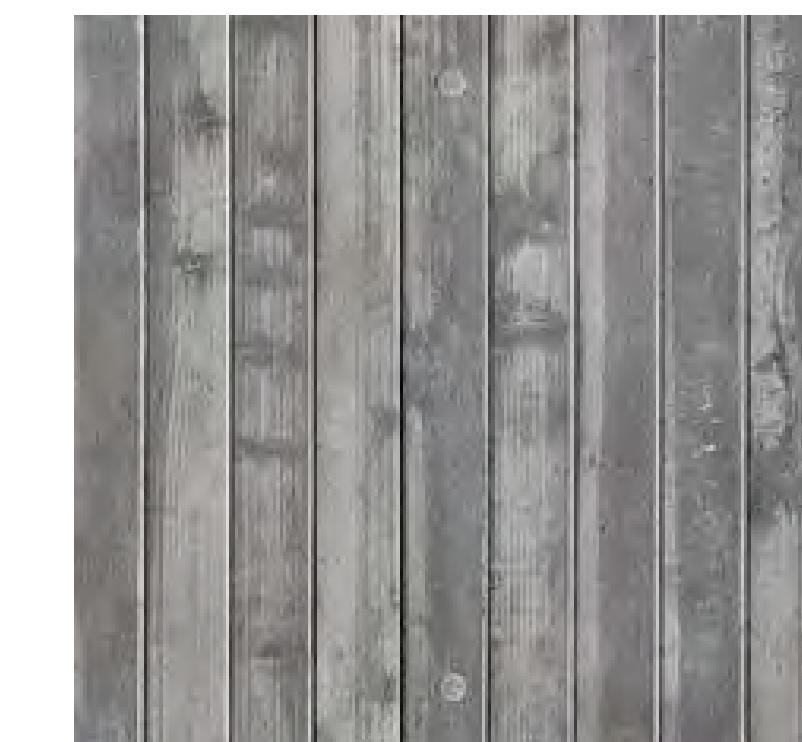
**D Vertical Board Formed Concrete**
