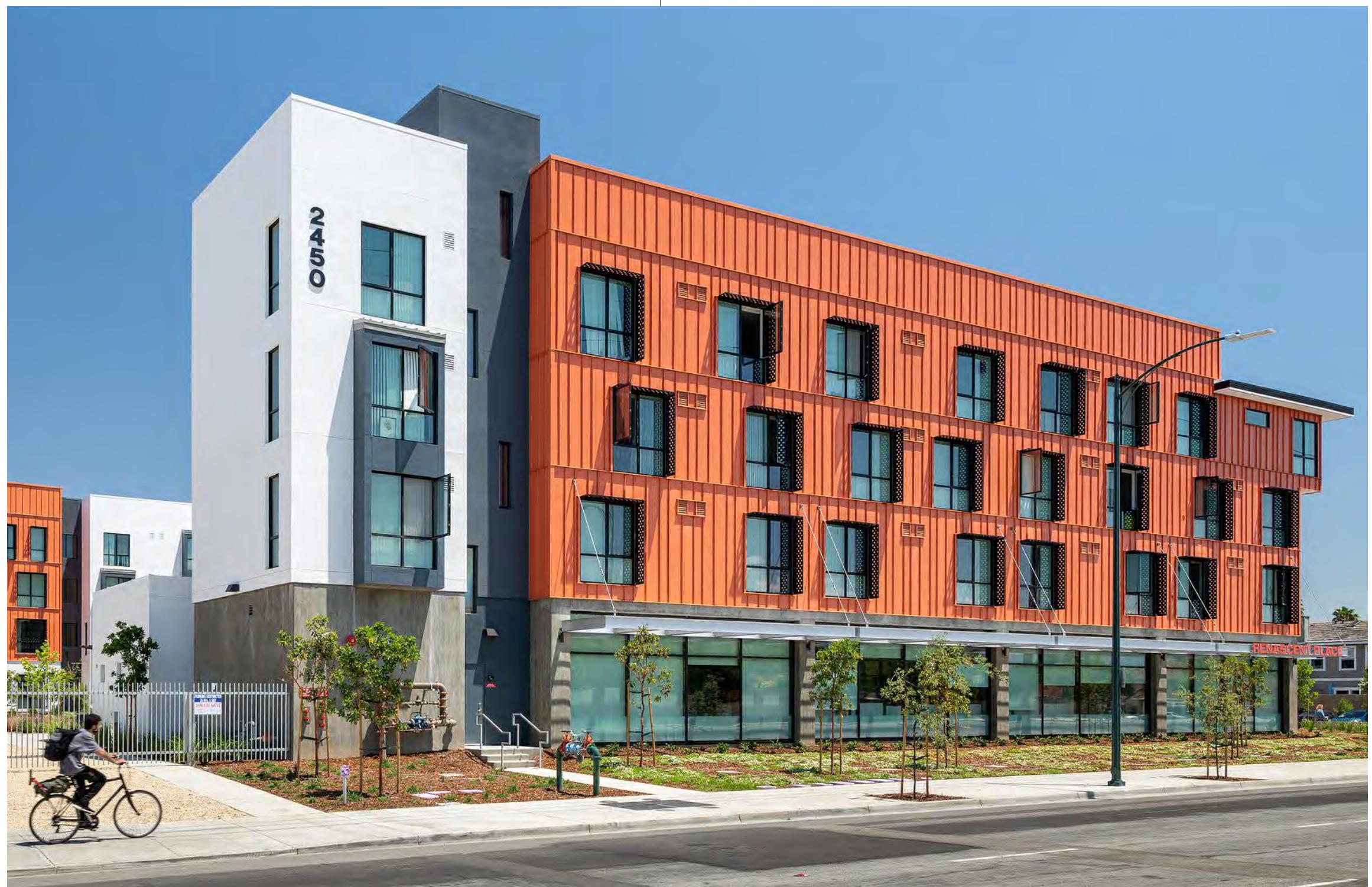
① Overall Example of Staggered Red Vertical Siding, White and Gray Medium Sand Finish Stucco
