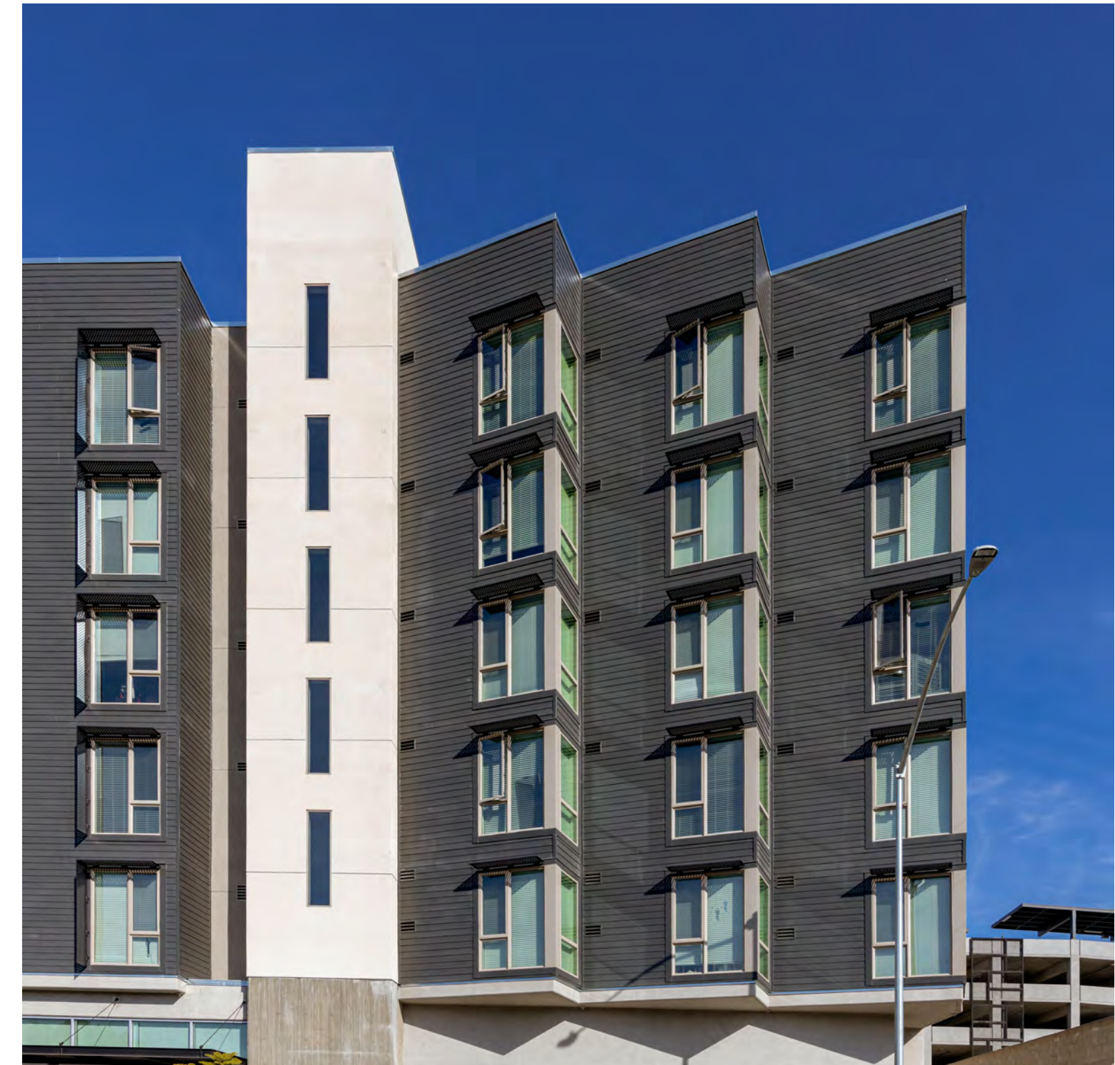
⑤ Example of Corner Bay Window Detailing with Gray Vinyl Windows, Lap Siding and Medium Sand Finish Stucco (Similar to North Elevation)
