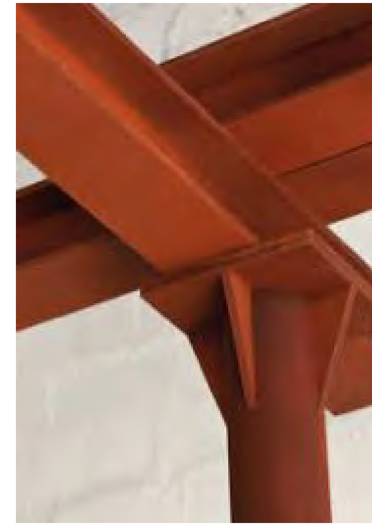
F Exposed Steel Trellis and Awnings Bonderized, Painted Similar to SW 6881 'Cayenne'
