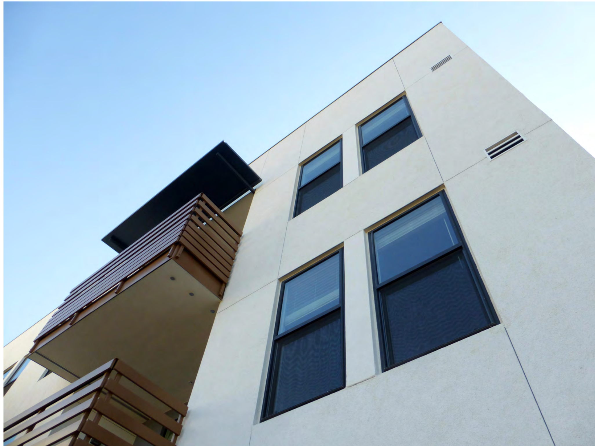
④ Recessed Single-Hung Dark Vinyl Windows in Medium Sand Finish Stucco Wall with Face-Mounted Balcony Guardrail (Basis of Design for Windows and Stucco Walls)
