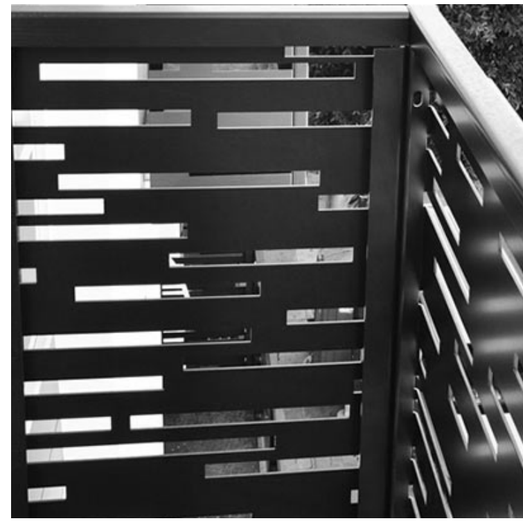
B Decorative Screen at Stairs and Parking Garage Similar to Bok Modern B14 or B21 Painted or Powder Coated Similar to SW 7675 'Sealskin'
