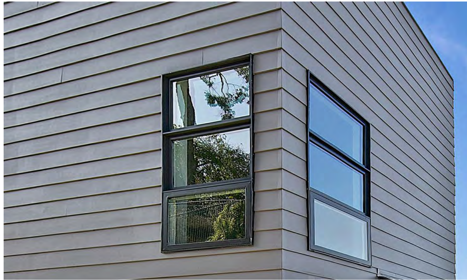
③ Example of Horizontal Lap Siding Steel Corner Cap (Flush window not indicative of intended alignment in lap siding)
