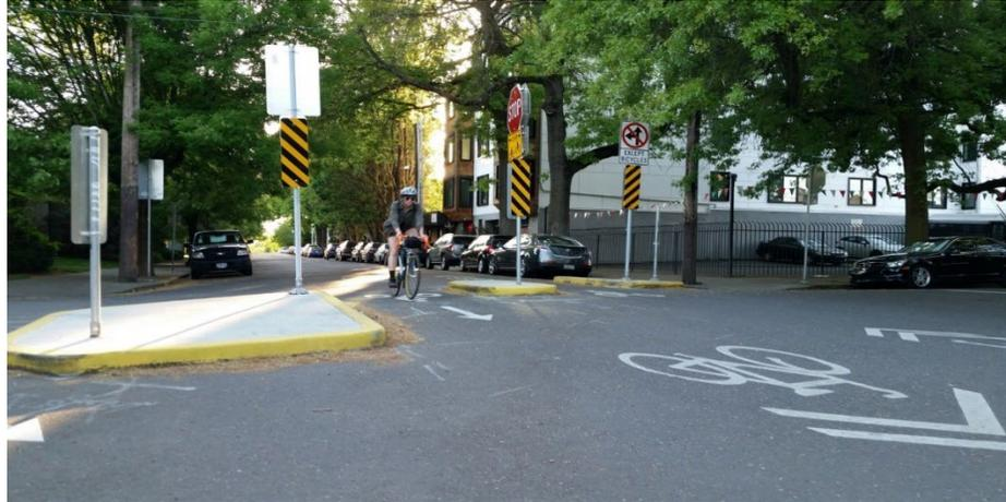
At intersections with larger roads, traffic diverters and enhanced crossings maintain connectivity for vulnerable roadway users and maintain low traffic volumes by discouraging or restricting cut through motor vehicle traffic. Bioswales and landscaping amenities enhance water retention capabilities and shade.
