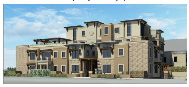
Exterior materials consist of stucco and stone in a warm natural palette. Accents include wood trellises and corbels stained in a rich medium brown tone, as well as metal deck railings. The roof material is proposed to be standing seam metal in a medium gray color. Proposed fencing is a mix of wood and wrought iron. A sample elevation is provided below.
