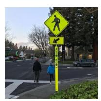
Example of sign post panel reflector installed at an uncontrolled, marked crosswalk location on Sylvan Avenue
