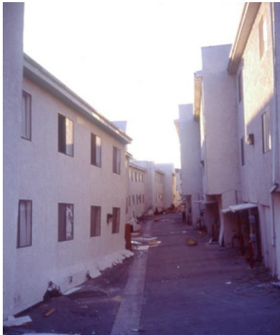
Left: Collapse. Right: Sidesway damage, Los Angeles, Northridge earthquake (Credit: Gary D. Avey)
