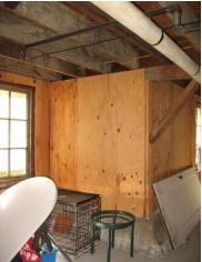
2A. Wood sheathing applied over existing studs, using the existing concrete foundation
