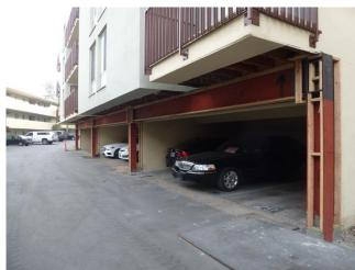
2C. Three-bay steel moment frame installed around garage door openings, with new concrete footing (Credit: Degenkolb Engineers)
