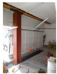
2D. Cantilever column installed with new concrete footing (awaiting concrete) (Credit: Thor Matteson)
