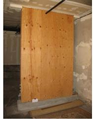
2B. New stand-alone wood shear wall with new concrete footing
