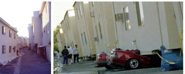
1C. Left: Collapsed 3-story building. Right: Sidesway damage, Los Angeles, Northridge earthquake (Credit: Gary D. Avey)
