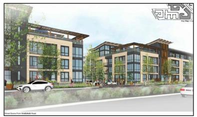
five-story structure with a maximum height at 58'. Similar to Building B, portions of this building near the entrance courtyard are stepped down to three stories with a maximum height of 38'.
