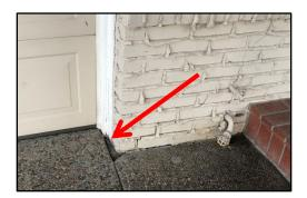
• The porch has been overlaid with a brick veneer and a section appears to have shifted, creating a lip and crack between the support post and the wall. Staff suspects that this could be a root issue but could also be a part of the construction detail or settling of the area. Again, the porch area near the post could be excavated to see if roots are impacting this location. (See photo below.)
