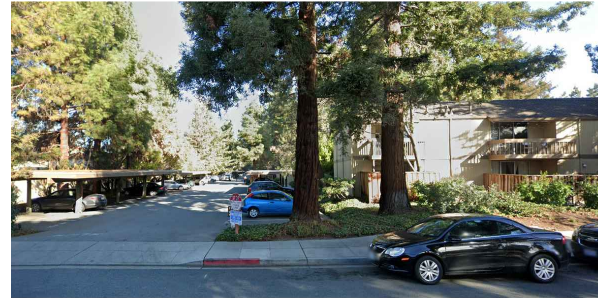
④ 225 - 236 CENTRAL AVENUE
