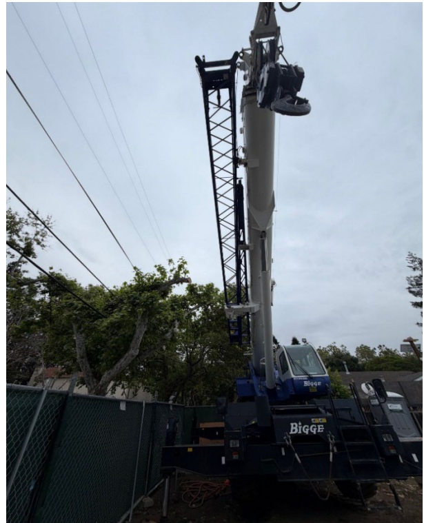
Photo #6 Photo of crane used to build home
