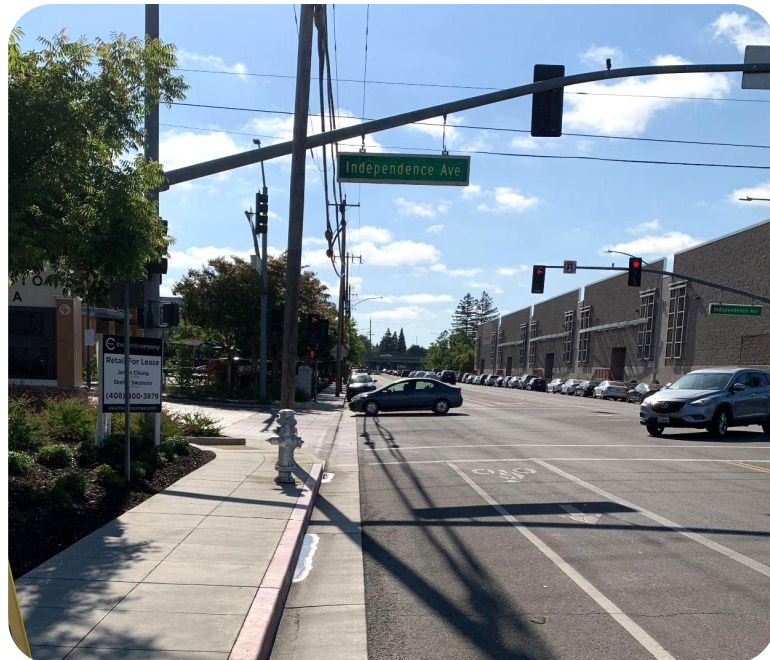
E. Charleston Road existing conditions (4' sidewalk)
