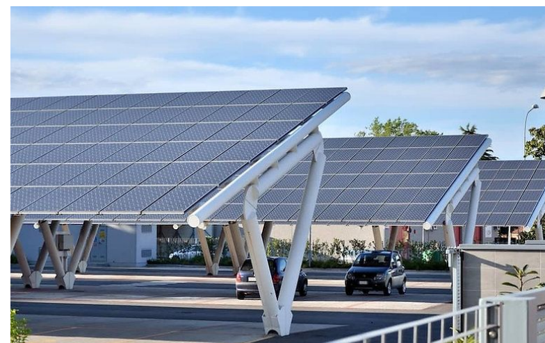
Rooftops will house solar panels to power a significant portion of the development.
