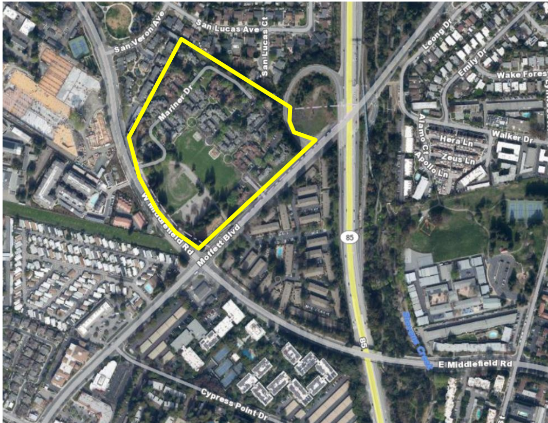
Figure 5: 500 Moffett Boulevard (Shenandoah Square Property)
