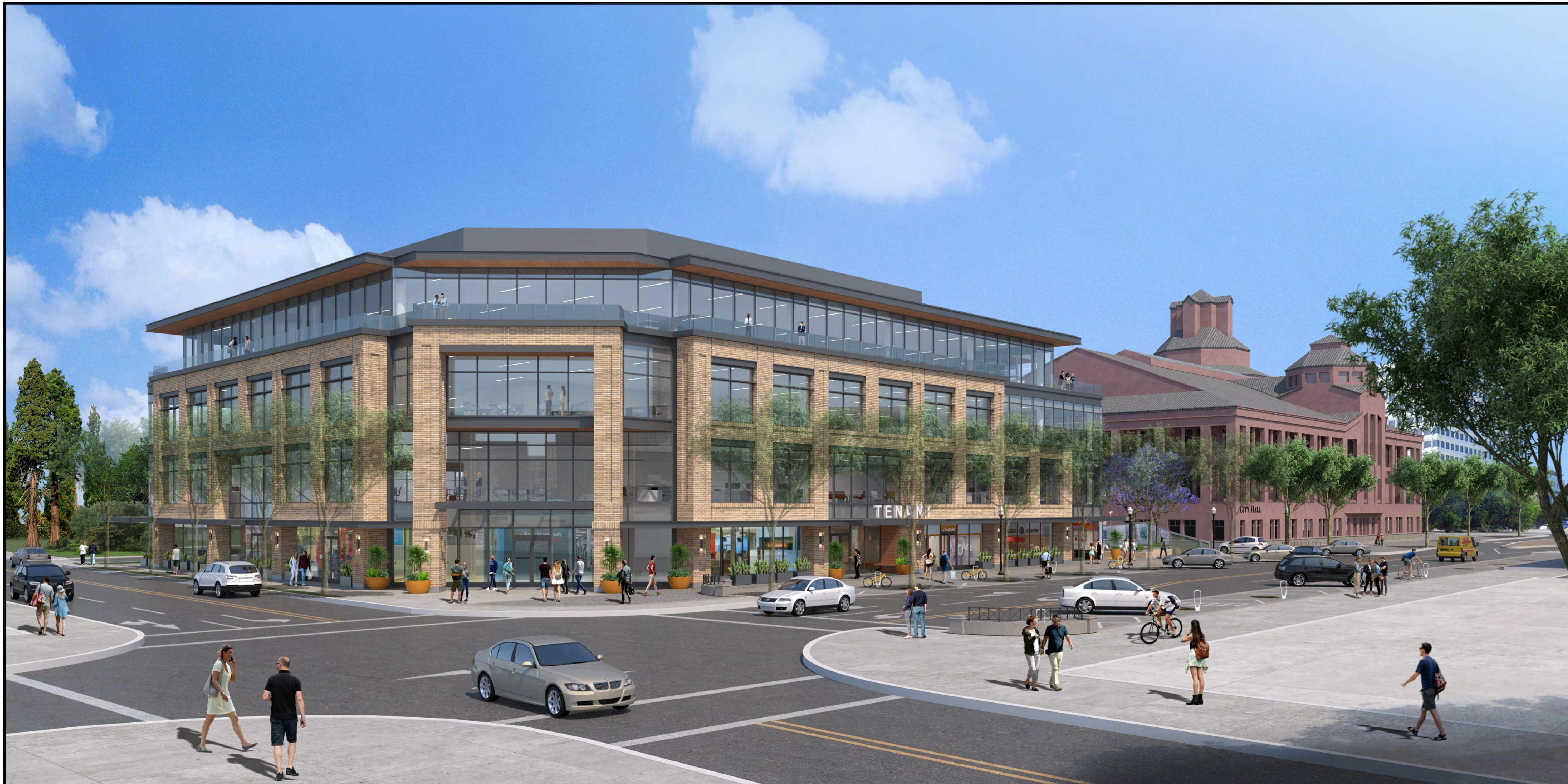
VIEW FROM CORNER OF CASTRO STREET & CHURCH STREET
