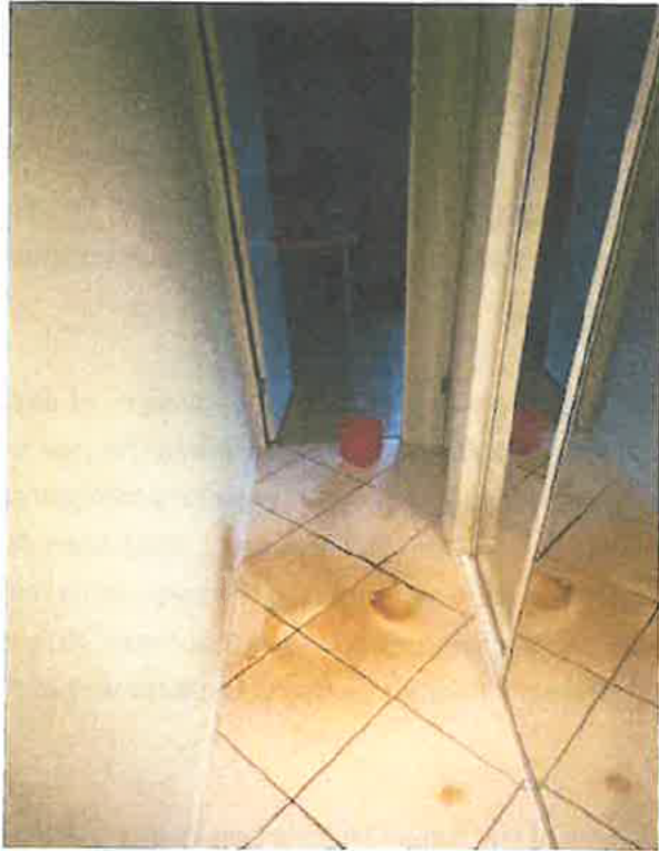
f. Homeowner Photo 2: interior view of roof leakage in southeast corner of home after rain. Please note the moldy skylight.
