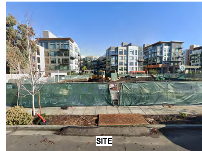
F) EXISTING SITE LOOKING EAST
