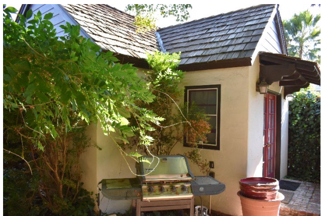
Figure 14. Context view of the rear ADU, looking northeast.
