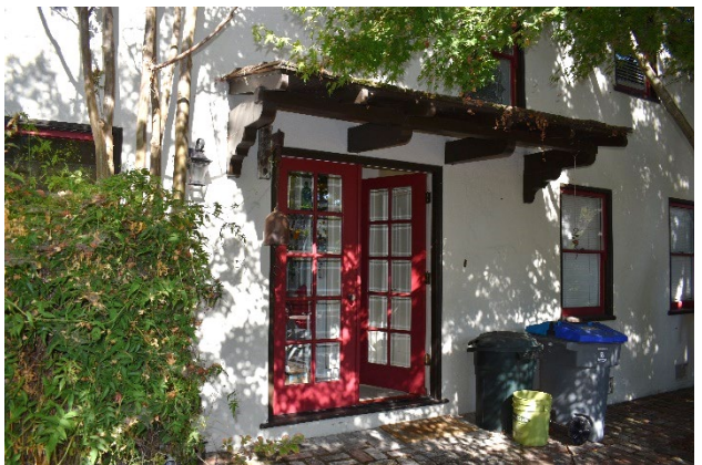
Figure 8. Rear façade, including a non-original French door, looking north.
