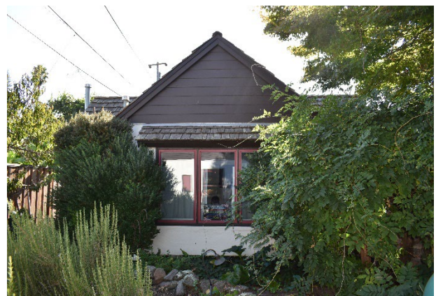
Figure 15. Side façade of the rear ADU, looking east.
