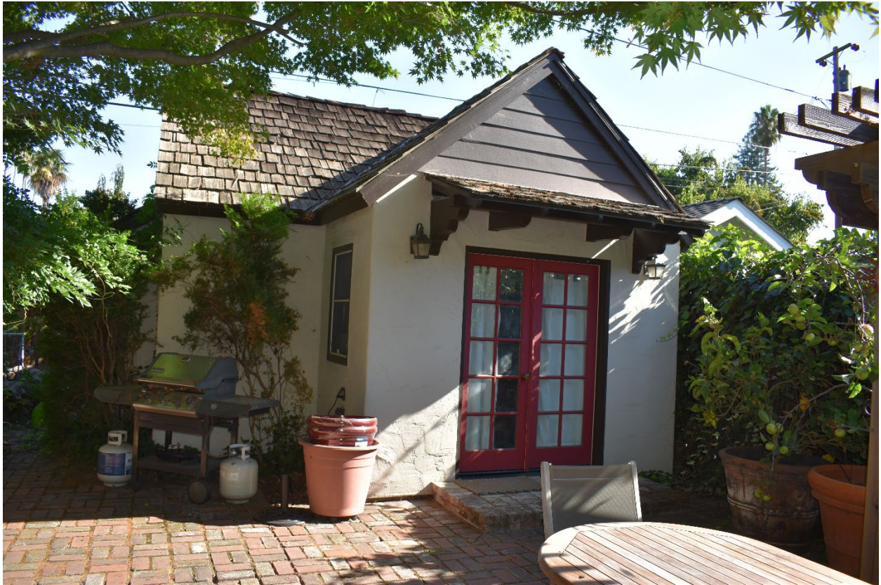
Figure 13. Context view of the rear ADU, looking northeast.
