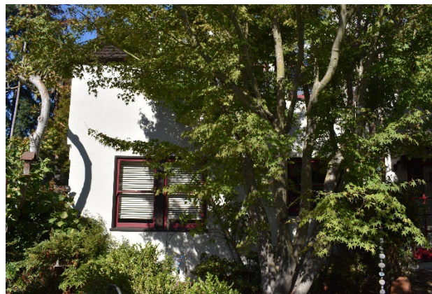
Figure 9. Fenestration along the southern side of the rear façade. Looking west.
