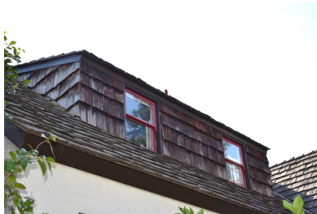
Figure 5. Detail view of west façade dormer, looking southeast.
