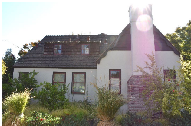
Figure 4. West façade, looking east.
