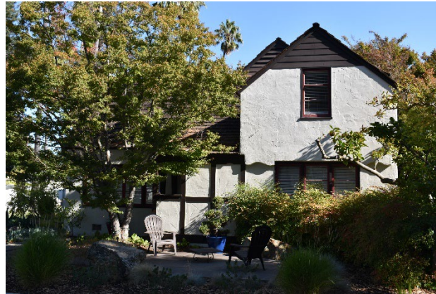
Figure 3. South façade, looking north.
