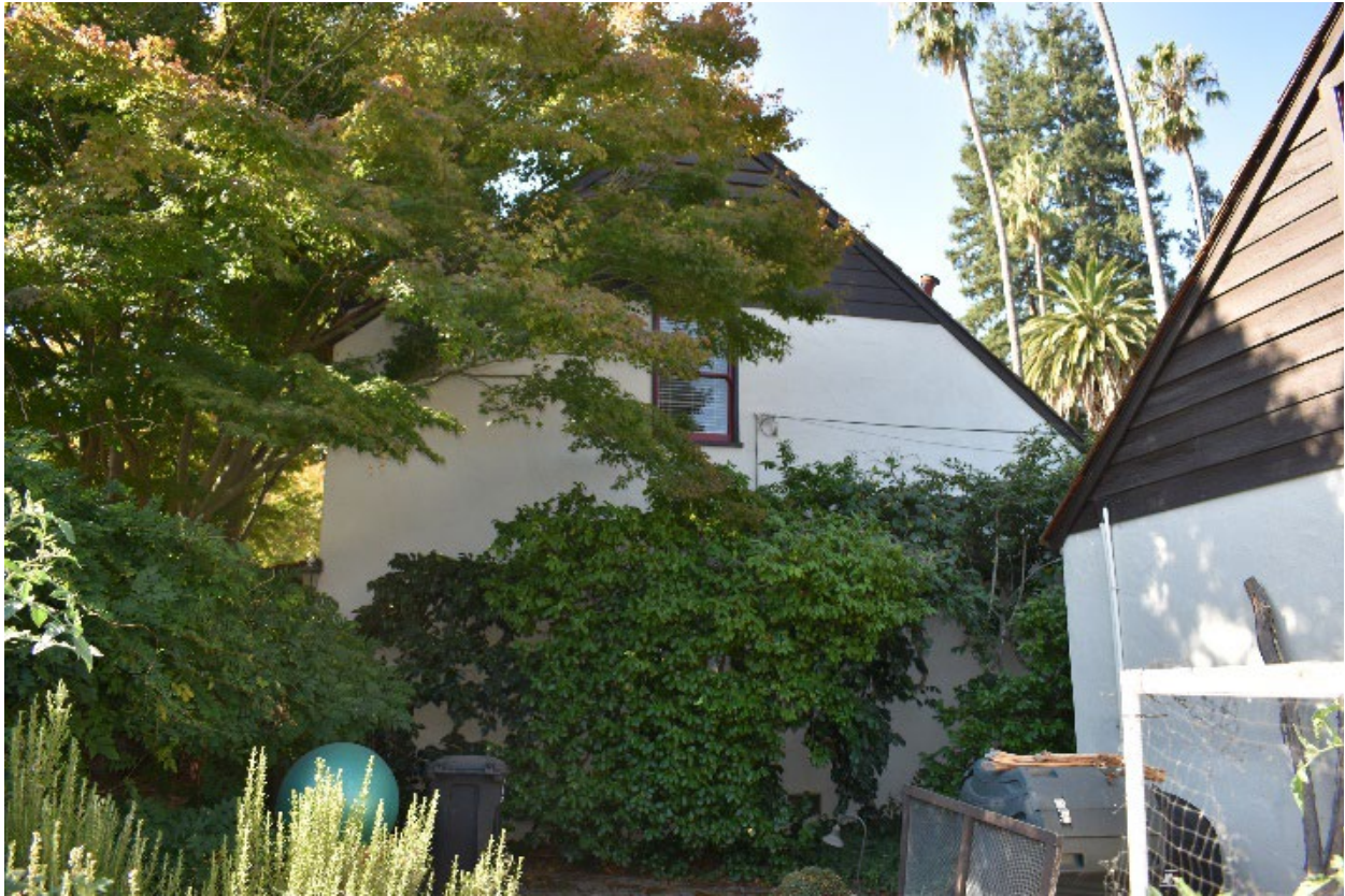
Figure 6. North facade, looking south.
