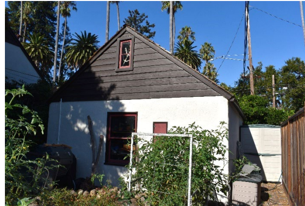
Figure 11. Rear façade of the garage, looking west.
