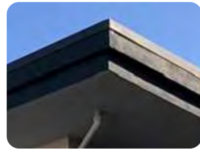
PAINT ROOF OVERHANG
