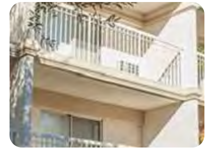
EXISTING BALCONY RAILINGS
