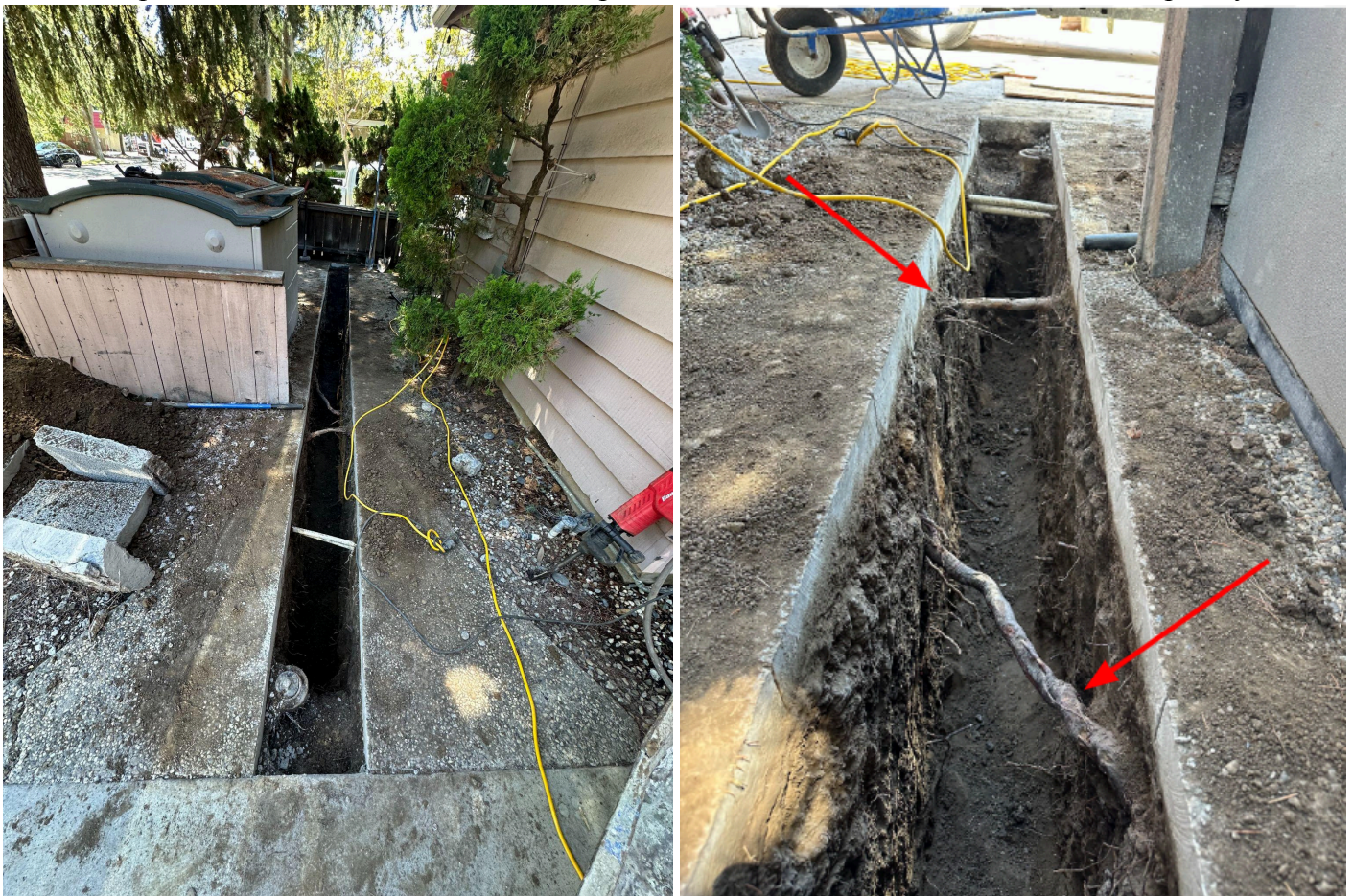
Showing the trench (left), showing only two roots encountered (right)
